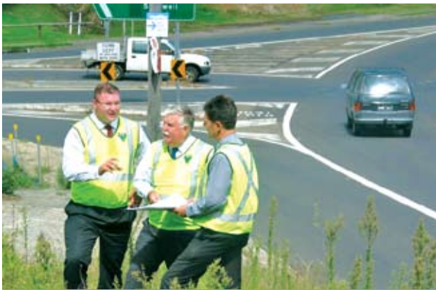
Paul inspecting progress on the Bulli Overpass with David Campbell, Minister for the Illawarra, and Stephen Arnold, RTA Southern Regional Manager.
